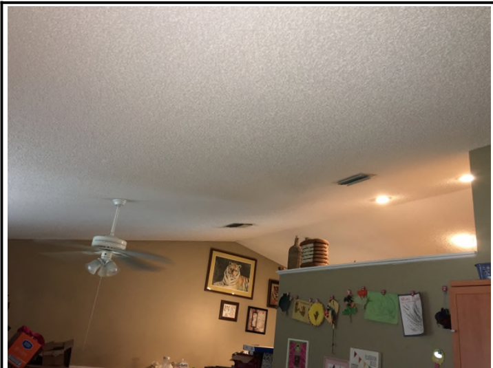
Good condition / no signs of leaks
