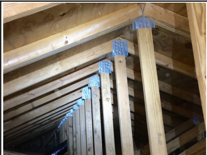
Good condition / no signs of leaks
