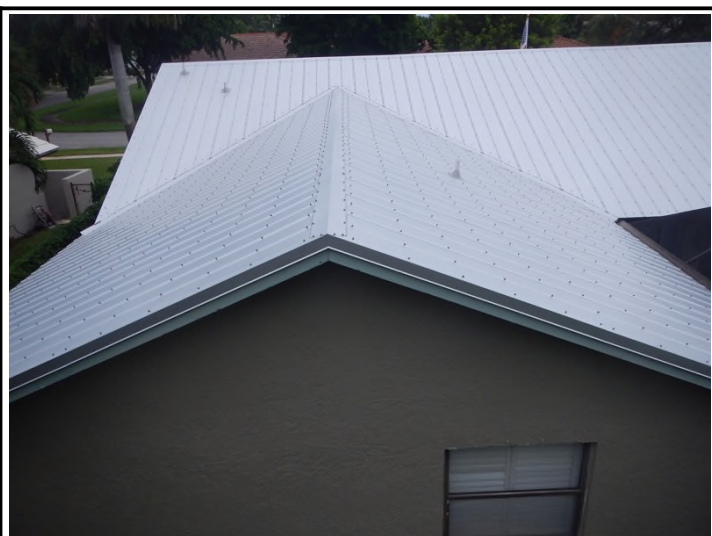
Seamless metal / good condition / 40 yrs remaining life
