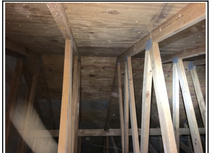
Good condition / no signs of leaks
