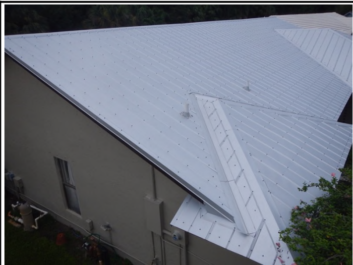
Seamless metal / good condition / 40 yrs remaining life
