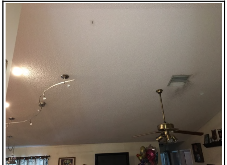
Good condition / no signs of leaks
