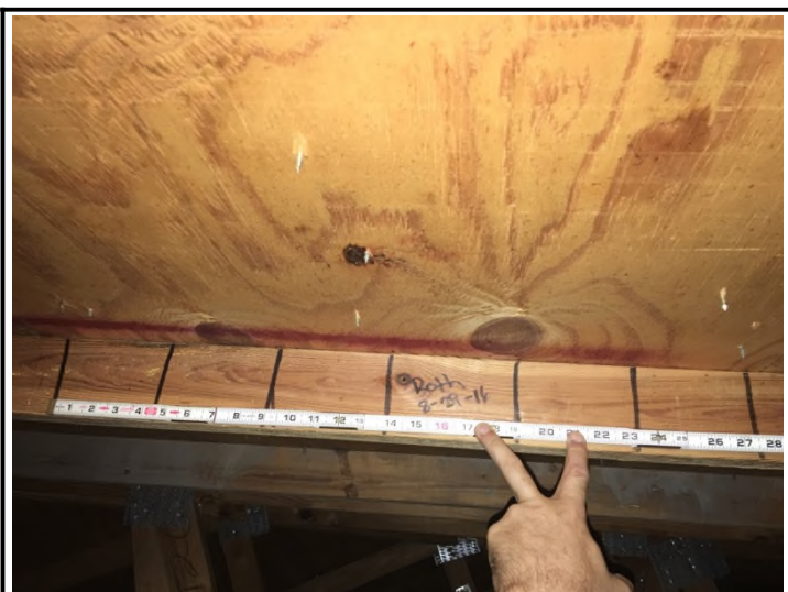
8d nails spaced 6" or less in the field
