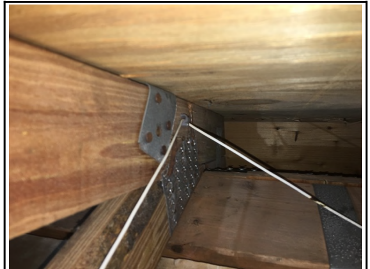
Single wraps (4 nails on opposing side)
