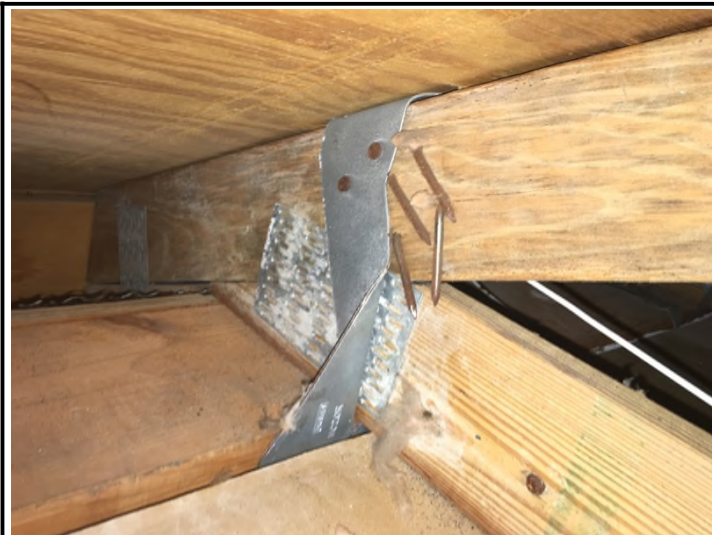
Single wraps (2 nails on truss face)
